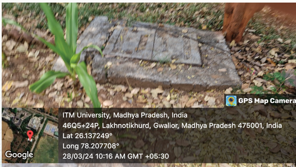
Septic tanks at various places in campus
